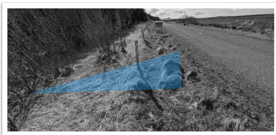
Figure 2.5 – Steep Approach Gradient Where Site Access E Connects to the L6309
